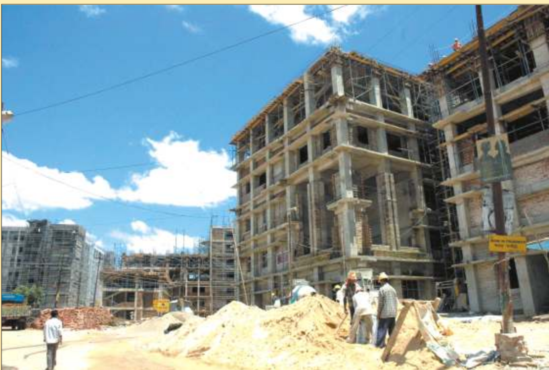
Construction work at Agartala Govt. Medical College
